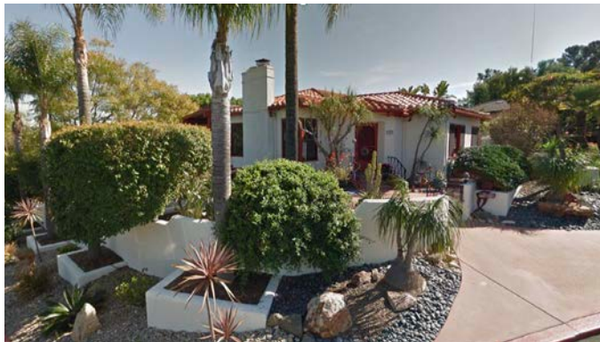
James & Corrine Dall House, built 1938.
